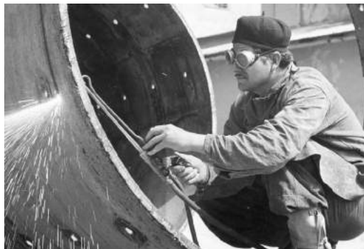
Disposal of the material mill in the old cement plant
