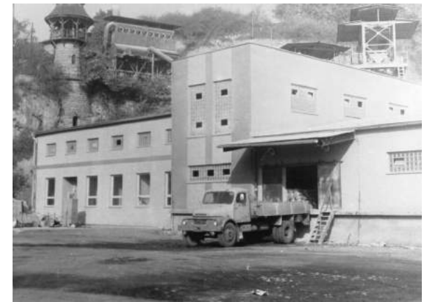
Mortar works in Srbsko
