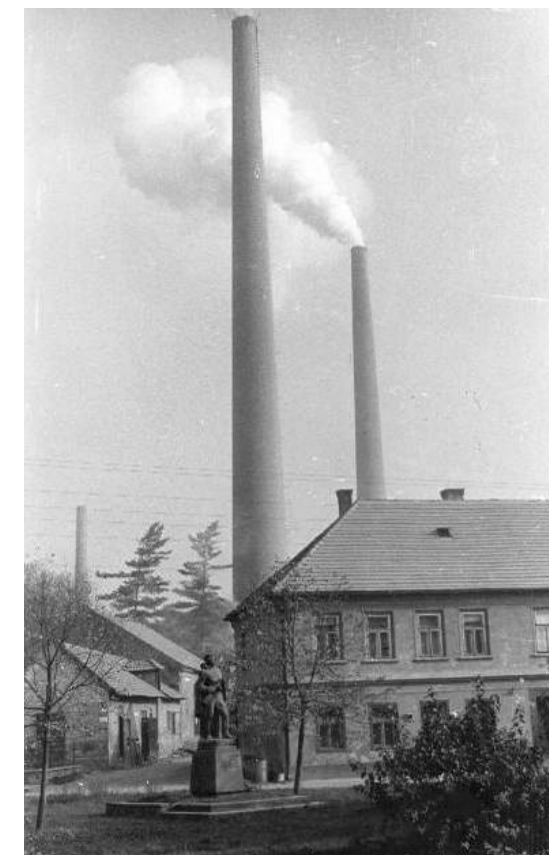
The old cement plant in hot commission
