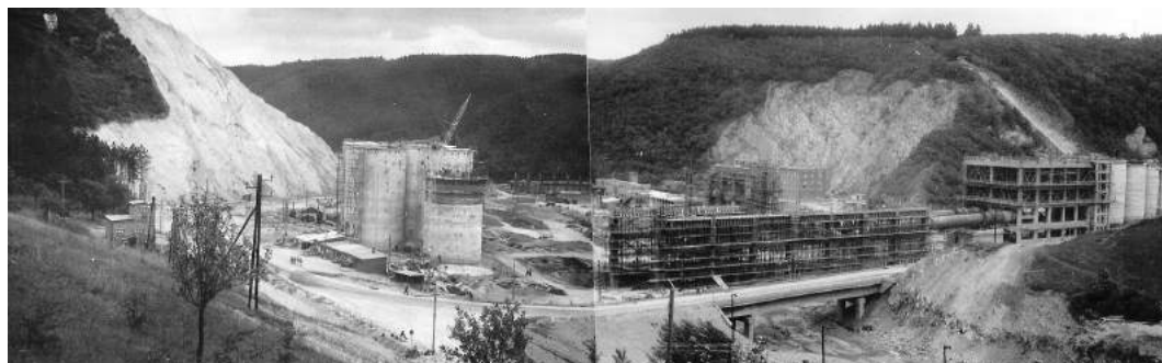
Overview of the cement plant construction
