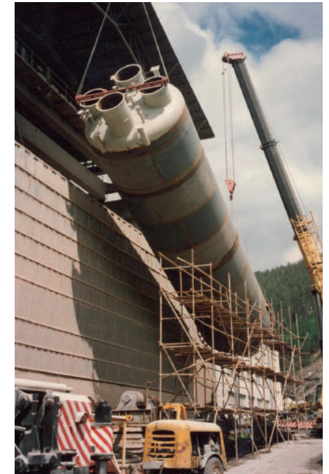
Construction of the coal mill
