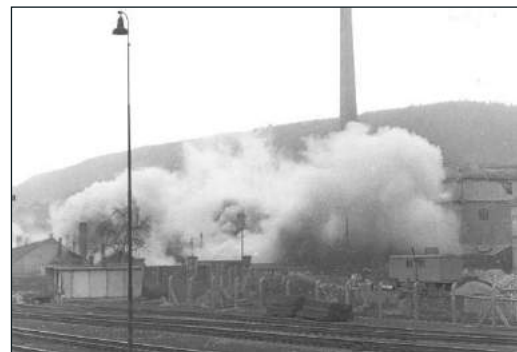
Demolition of the old cement plant
