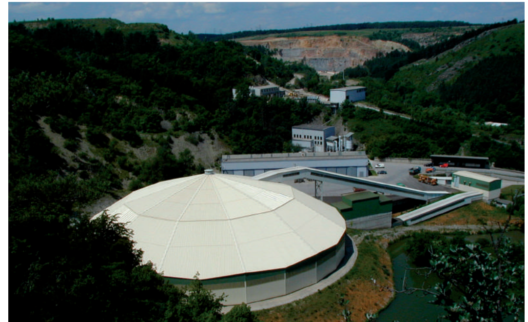
View of the PHS from a water works to the quarries
