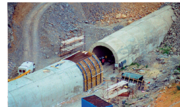
Prolongation of the tunnel to 332 meters
