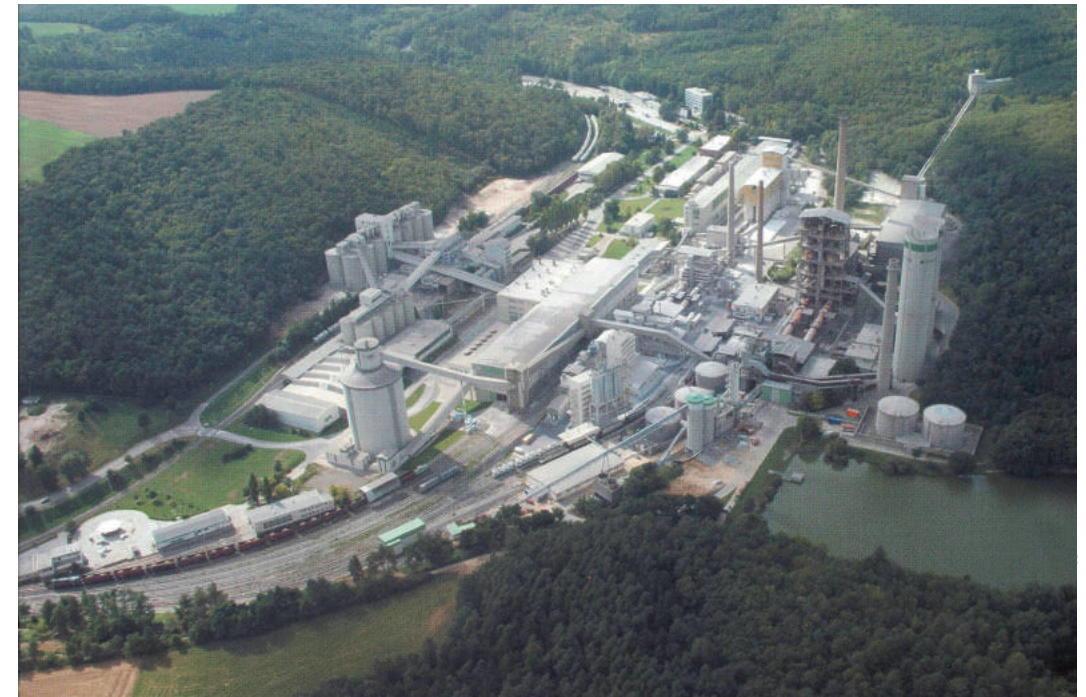
The Mokrá Cement Works
