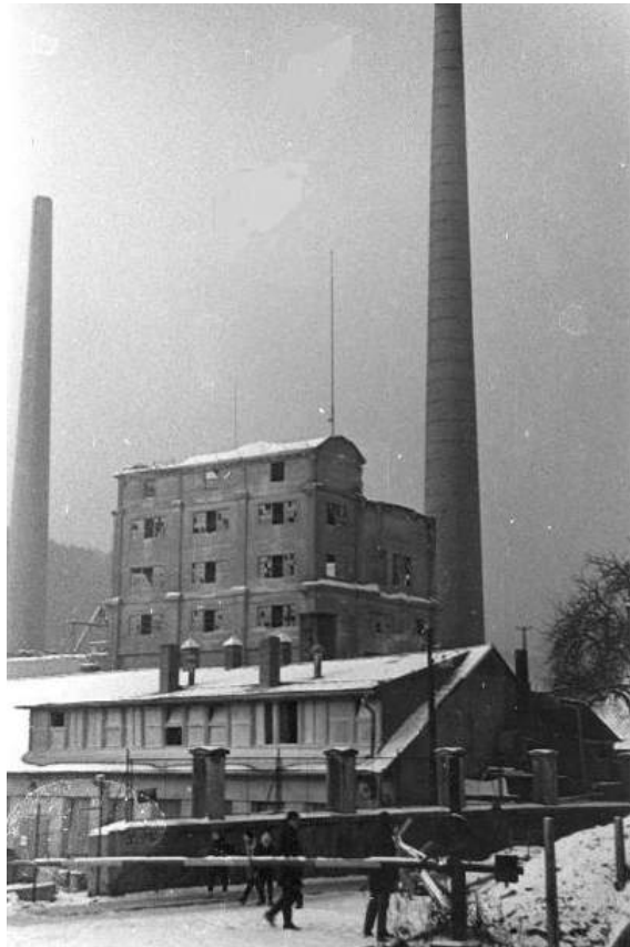
The old cement plant from the railway crossing
