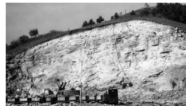
Loading raw materials on carriages of the narrow-gauge track
