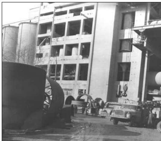
Repair of the rotary kiln jacket
