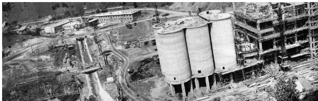
Construction of the new cement plant – material silos
