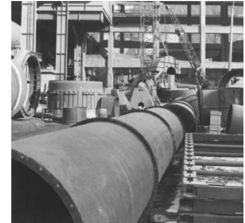
Repair of pipes running to the electric filters
