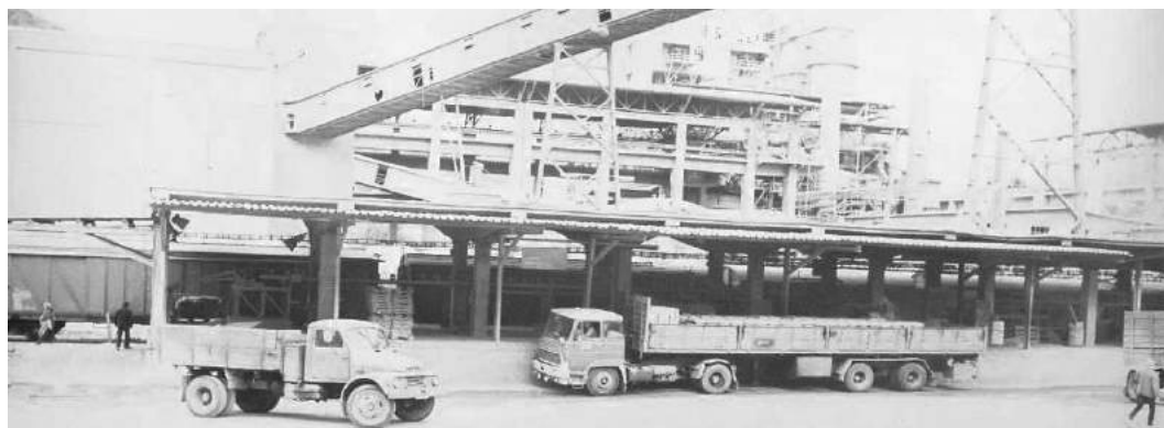
Dispatching of bagged cement
