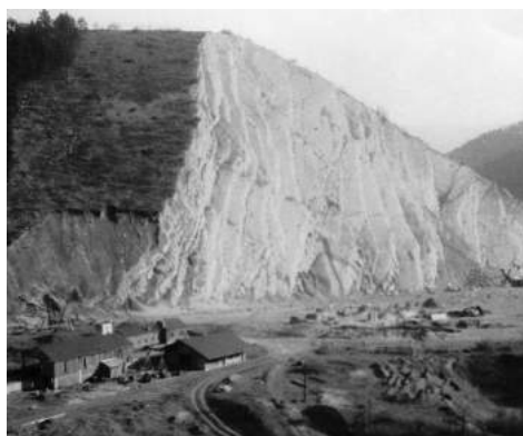
Space for a new cement plant
